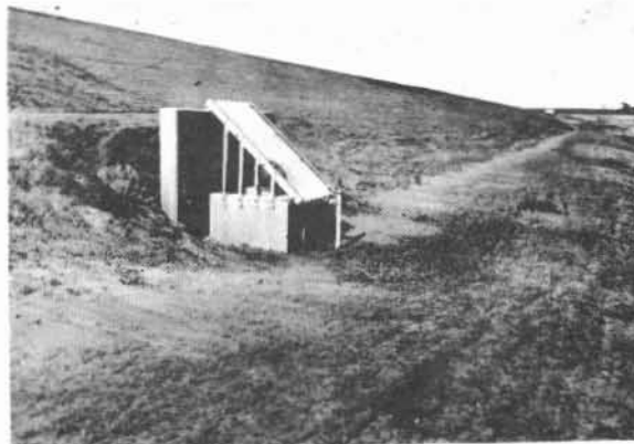
(b) Drop-outlet structure at subwatershed No. 1
