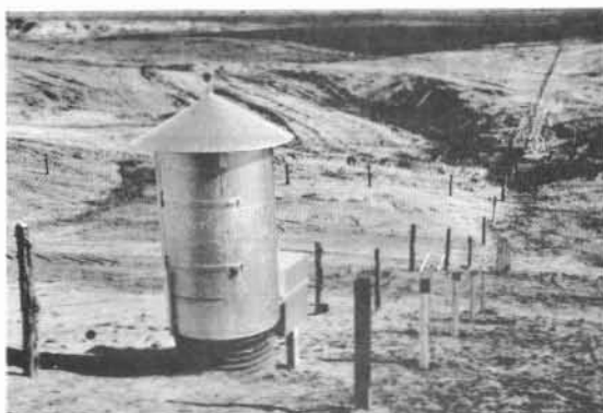
(c) Subwatershed No. 1 (after construction)
